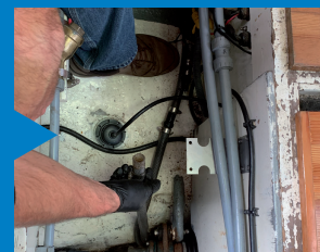
8. Showing the pipe from the bilge to connect into the Wavestream
