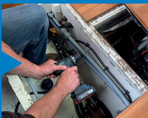
6. Drilling holes for mounting the bracket
