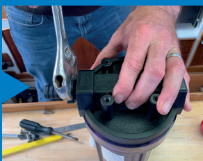
11. Ensure a tight fit for the connectors using a spanner
