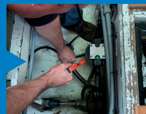
13. Cutting the bilge pipe to length
