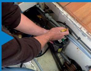
5. Marking holes to fit the bracket
