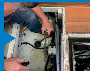
14. Fitting the outlet pipe
